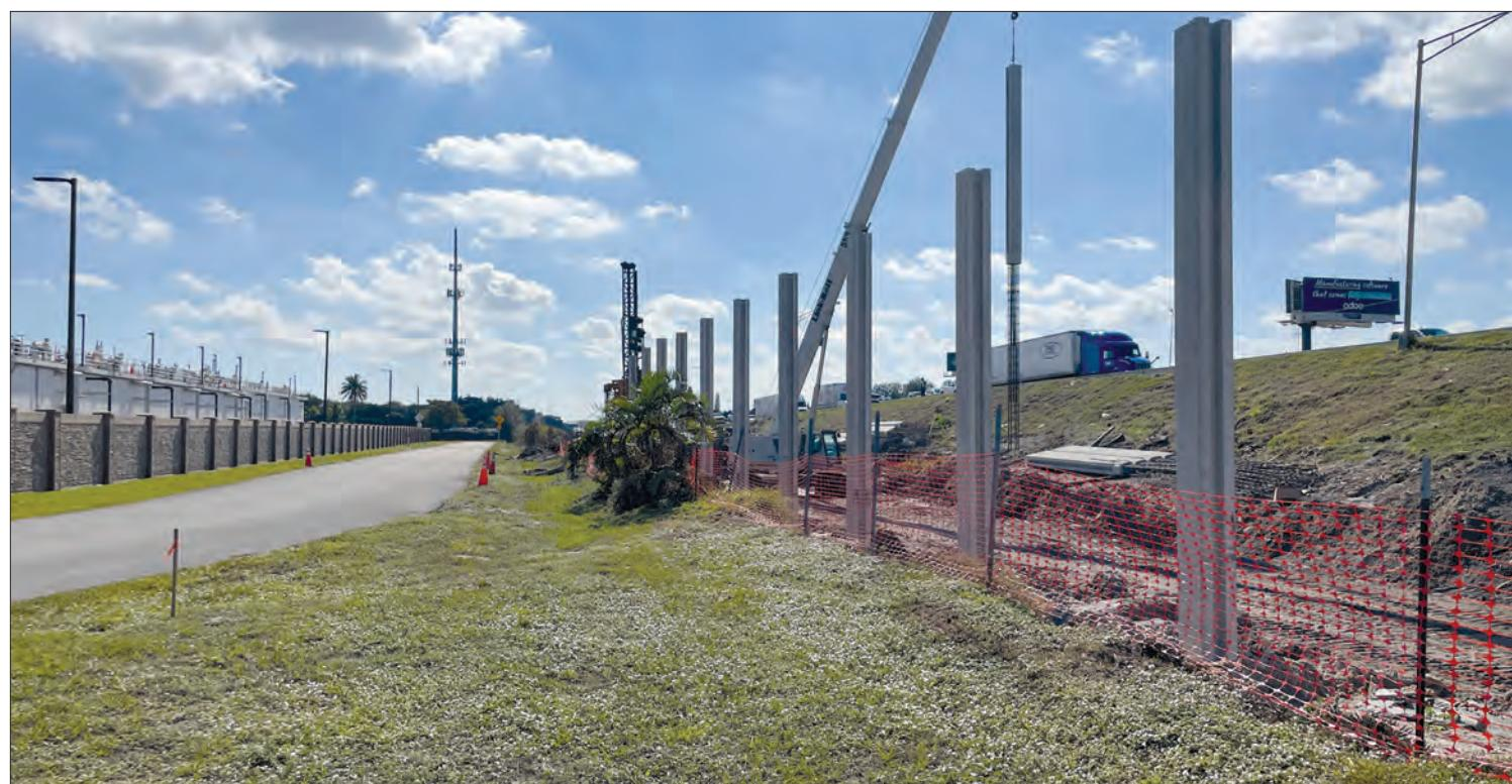
Construction of noise walls takes place between the northbound Florida Turnpike lanes and a Seminole Tribe Public Works facility on the Hollywood Reservation as seen on Dec. 5. Walls are also being installed along the southbound lanes in the back of tribal headquarters and tribal homes as Turnpike widening takes place in both directions.
