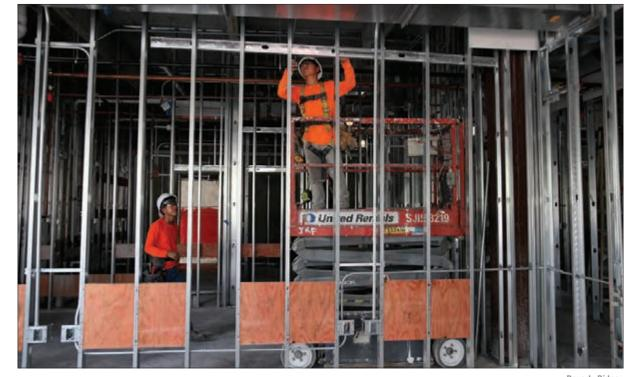
Workers construct the steel frame for walls on the ground floor administrative offices.
