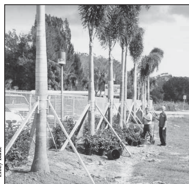
Newly planted palms require 2-by-4 reinforcement.
